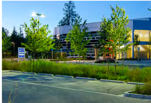
PARKING LOT AND PLANTED TRENCH
